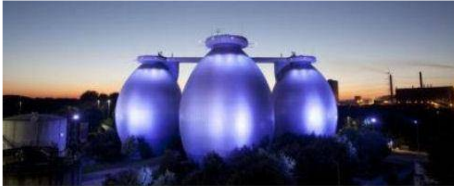
Figure 7: The Bottrop Wastewater Treatment Plant
