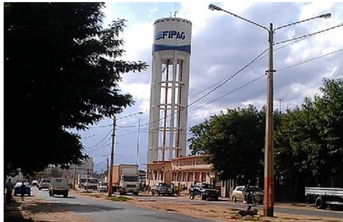
Figure 14: FIPAG Water supply tower
