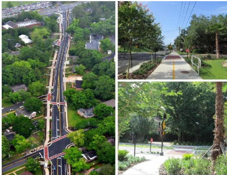
Figure 18: Franklin Boulevard after drainage Improvements
