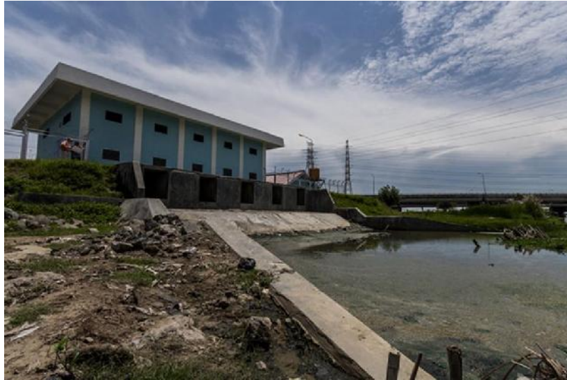
Figure 33: Semarang Polder pumping station
